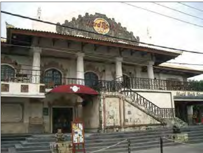
Bali (before renovation)
