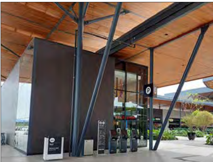
Florianópolis Airport Rock Shop (closed June 2023)
