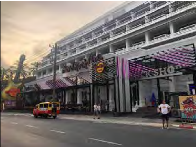
Phuket (new facade)
