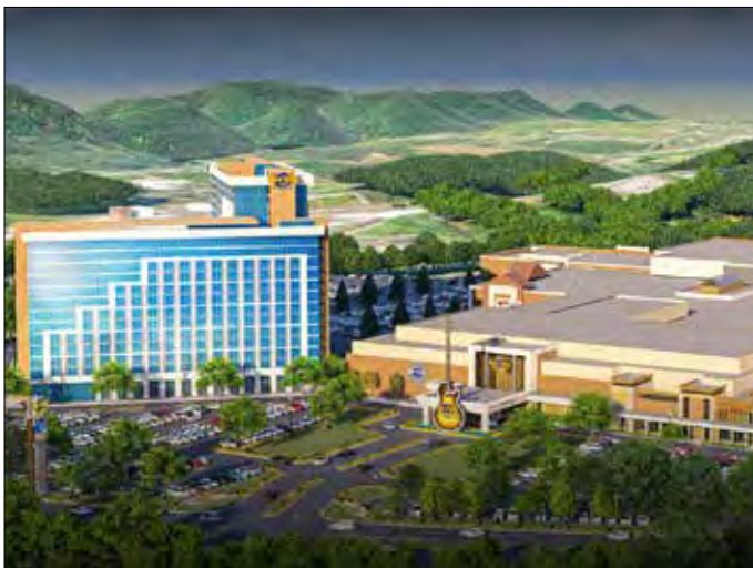
Bristol Hotel and Casino (opening 2025)
