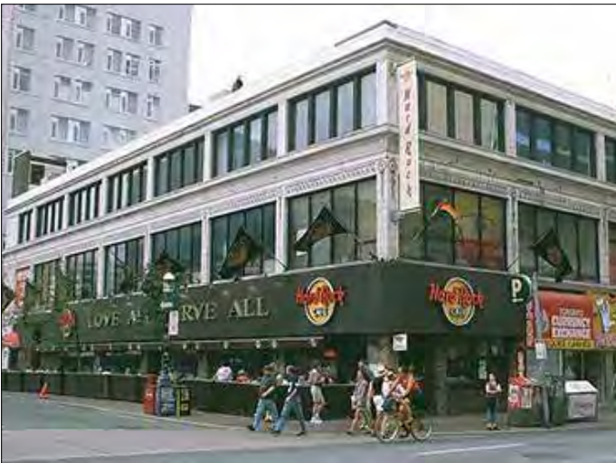
Toronto (old facade) (closed May, 2001)
