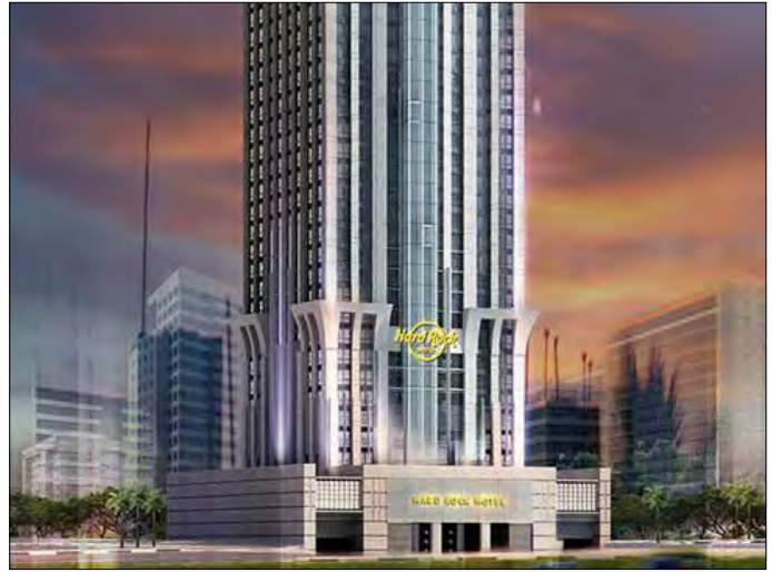
Dubai (project cancelled)
