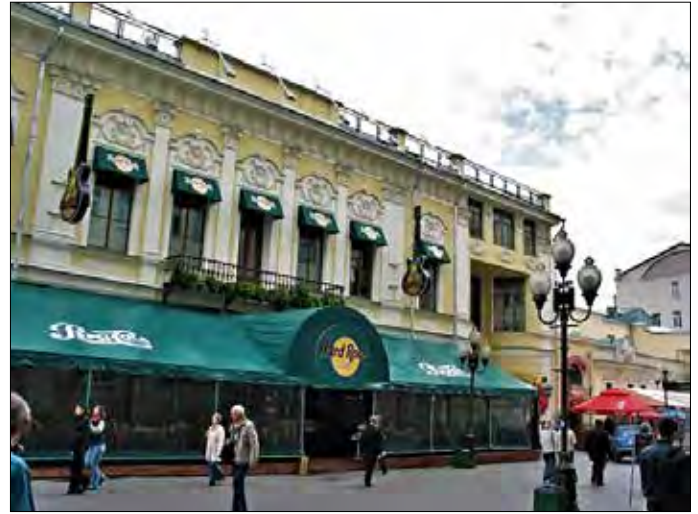
Moscow (different facade) (closed October, 2022)
