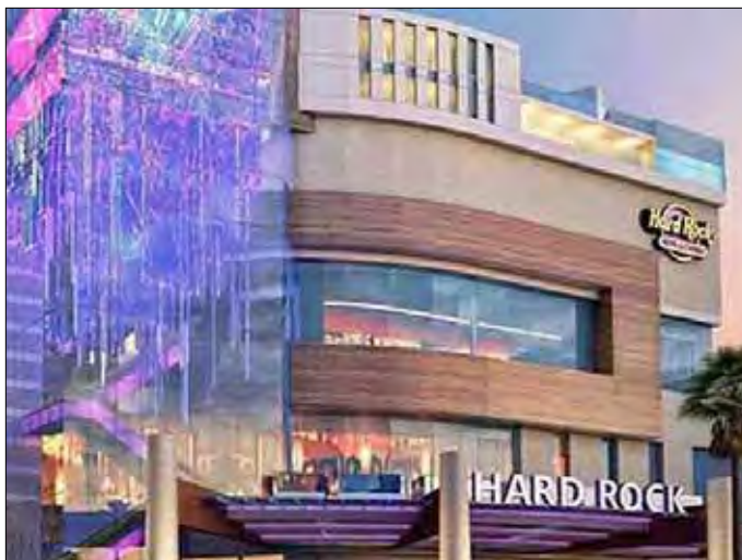
Santa Domingo Hotel and Casino (project cancelled. The plan was opposed by the community)
