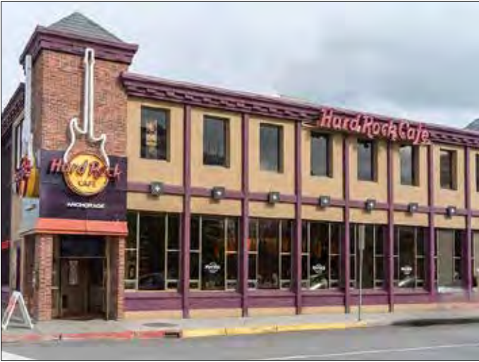
Anchorage (side view) (closed March 2020)
