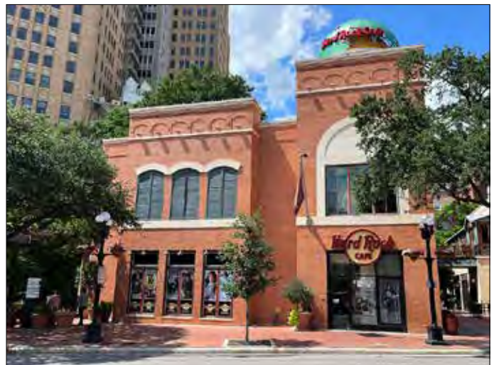
San Antonio on the riverwalk (new facade)
